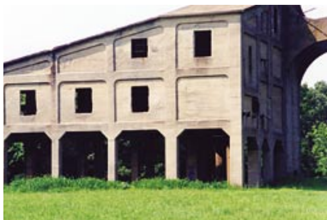
Fig. 3: After more than 80 years, the structure is still in excellent condition, having resisted decades of freezing and thawing
