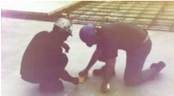
Fig. 3: Students scan and mark the concrete surface
