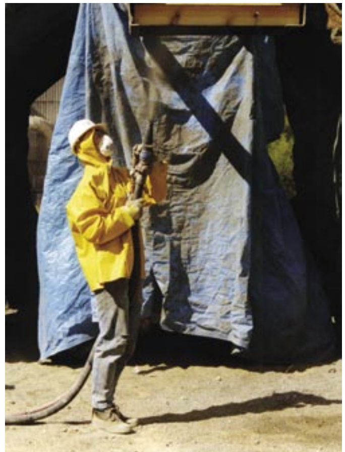
An ACI Shotcrete Nozzelman certification exam in progress
